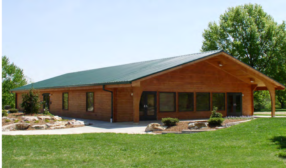
Riechmann Pavilion at Stephens Lake Park
