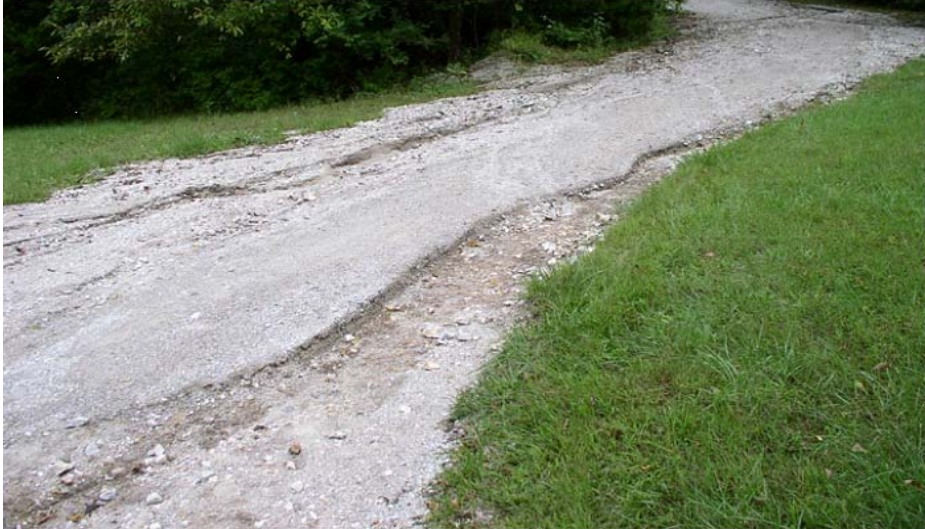
Bear Creek Trail washout after storm
