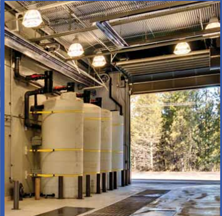
Town of Truckee Public Service Center Wash Bay & Rainwater Storage
