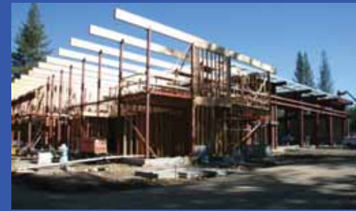
New Construction- Administration Building, custom wood framing; Maintenance Building, pre-engineered metal building
