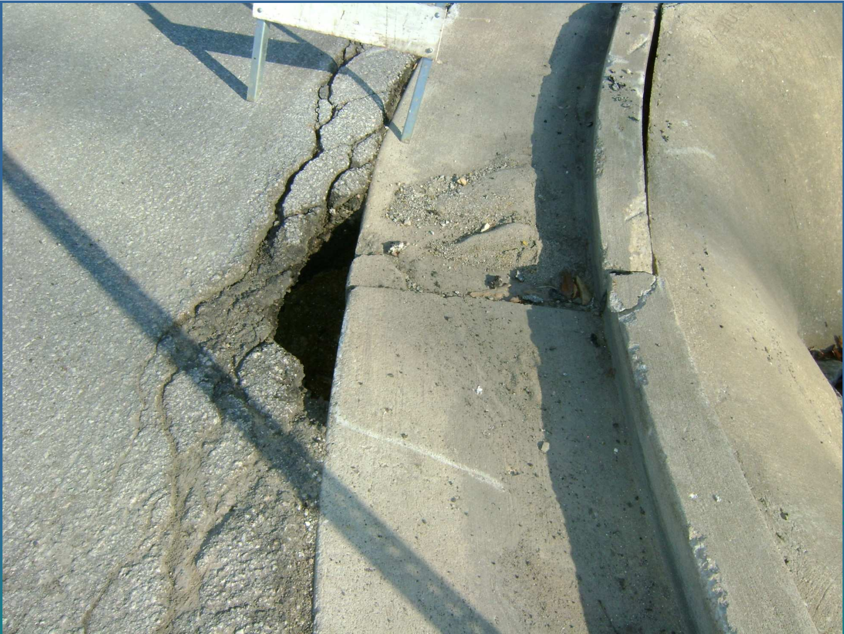
Jenni Lane Sinkhole due to failing storm pipe – still in service
