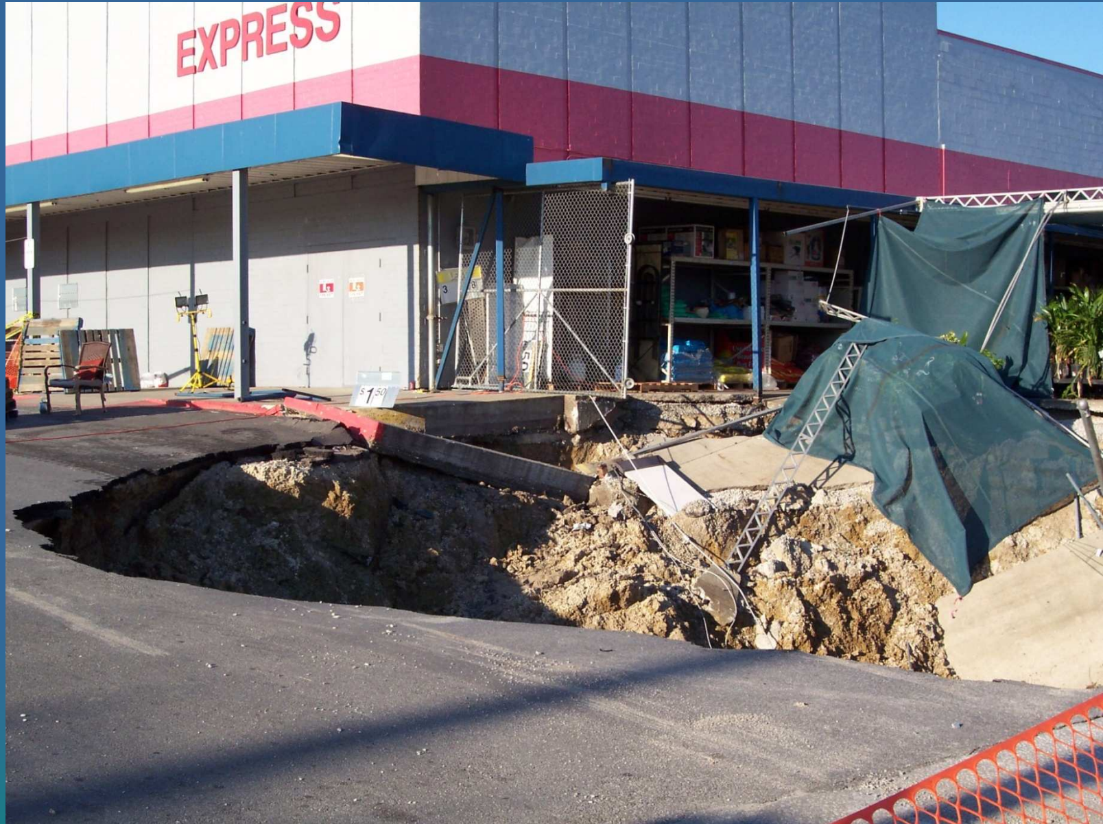
Worley & Stadium – old WalMart site Sinkhole due to storm pipe failure
