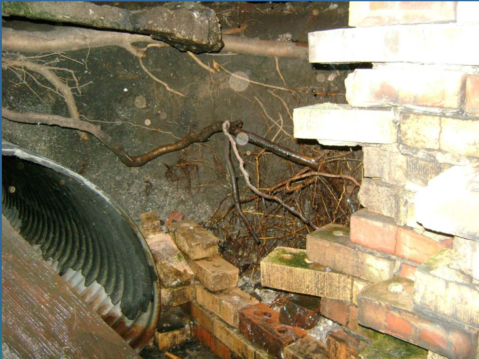
Worley Street at Health Department Failing inlet box – still in service
